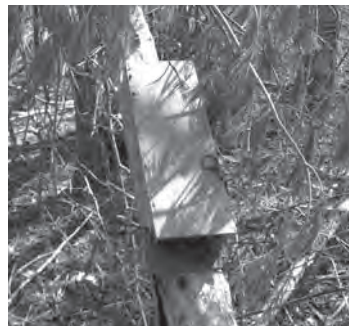
Leaning pole set
